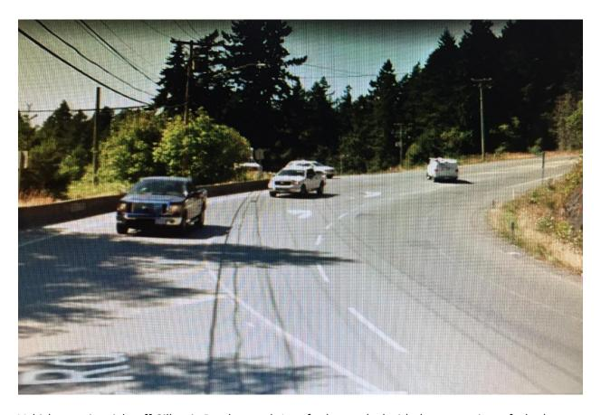
Vehicles turning right off Gillespie Road towards Langford must deal with the uncertainty of whether or not there is one or two (right and/or left) turning lanes, limited visibility due to the physical location of the junction at a curve in Highway 14, and the speed of oncoming traffic.
